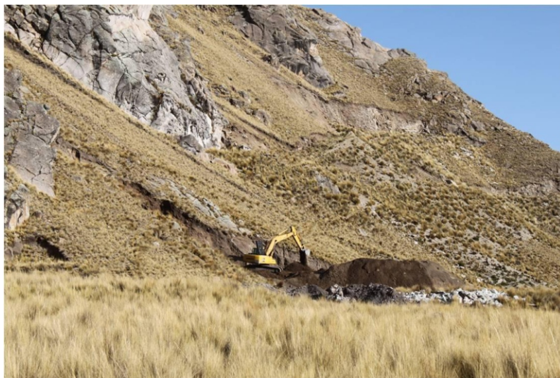
Figure 7. Stockpiling gold-bearing colluvium, southern flanks of Cerro Hemoso, Santa Barbara project
